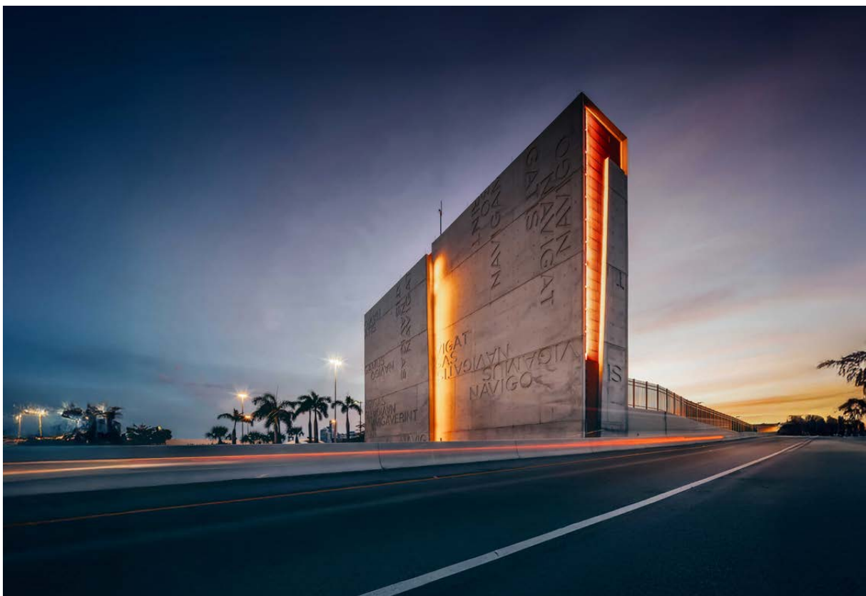
Port of Miami Tunnel, USA
