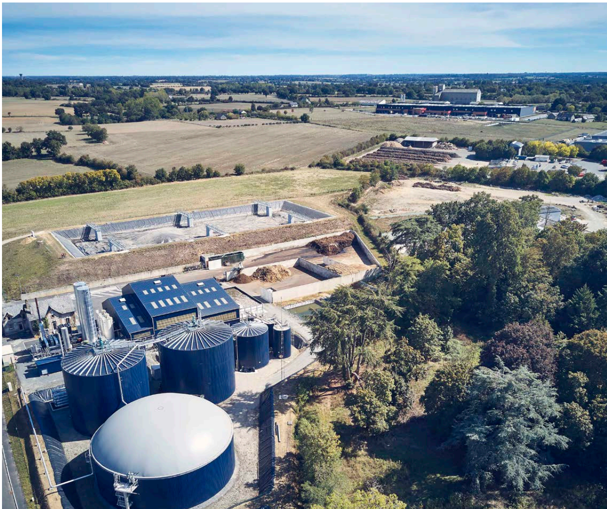
Evergaz biomass plant, Château Gontier, France
