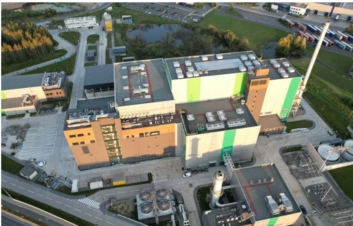
Olsztyn Waste to Energy Plant, Poland
