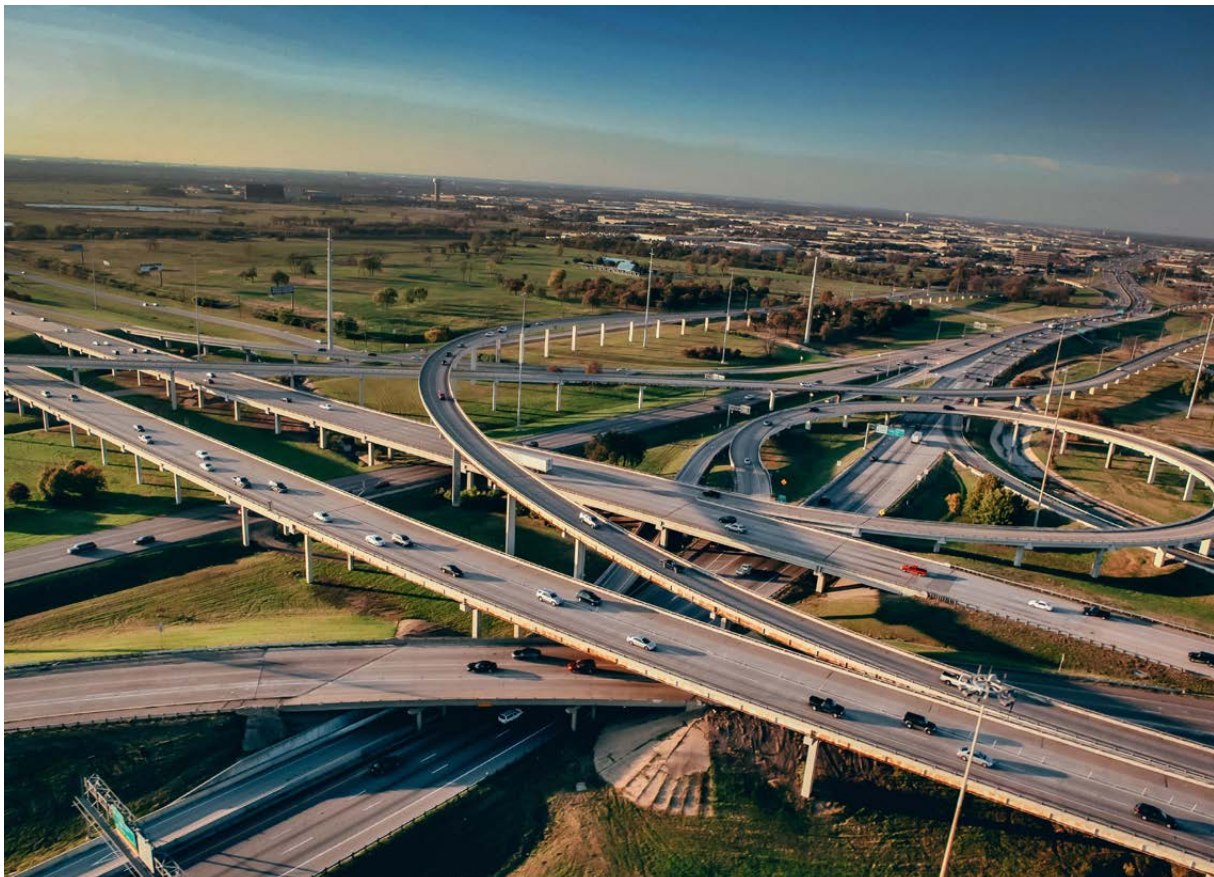
LBJ Express Highway – Texas, USA
