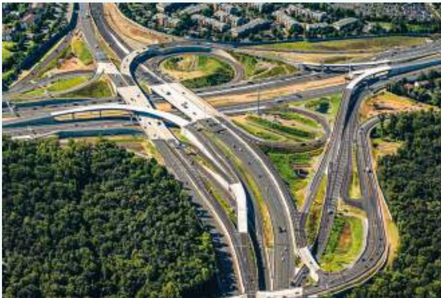
I-66 managed lanes, Virginia, USA
