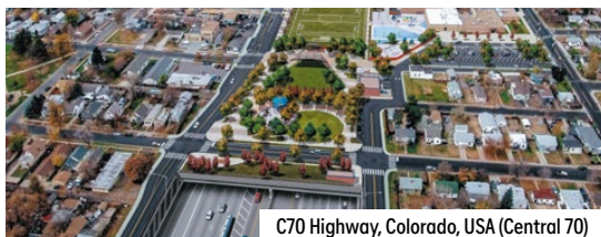
C70 Highway, Colorado, USA (Central 70)
