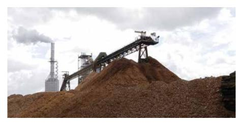
that supplies the presses. With a view to de-carbonisation, the use of the biomass unit will make it possible to **substitute much of the gas for biomass** - between **80 and 95**% for the entire site, depending on its level of activity, saving 35,000 tonnes of fossil fuel CO<sub>2</sub> emissions per year-in order to **produce renewable**, and green energy and reduce the site's ecological footprint.
