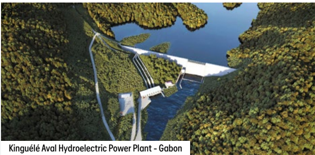
Kinguélé Aval Hydroelectric Power Plant - Gabon
