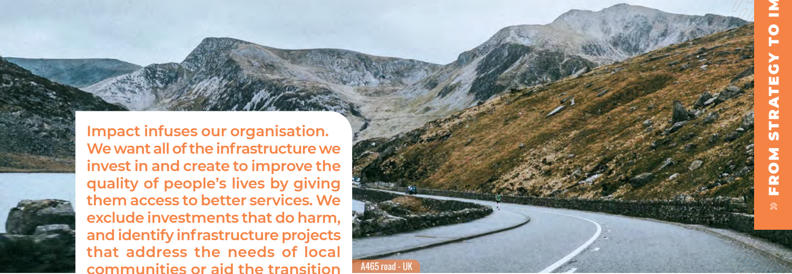
A465 road - UK
